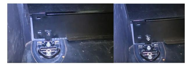
Center the wall with gaps on both sides and tighten, hold the wall level to the floor and tighten the carriage bolts. 10:10
